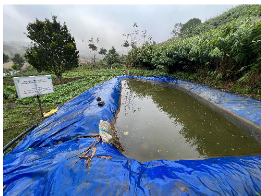
Low-cost water harvesting structure (Jalkund)
