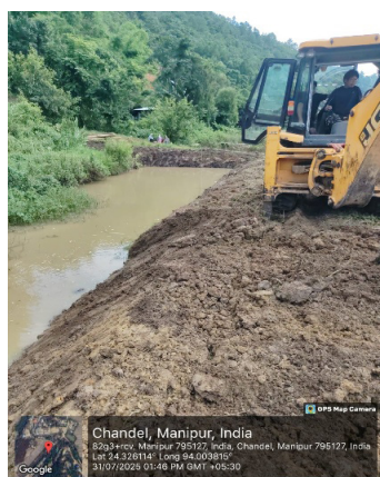
Renovation of farm pond
