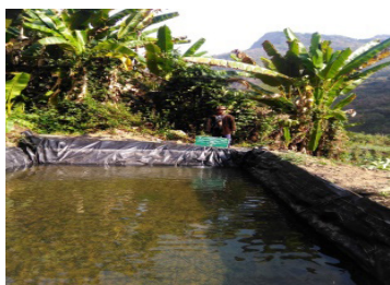
Low-cost rainwater harvesting structure (Jalkund) as lifesaving irrigation for Rabi crops
