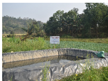
Low cost water harvesting unit
